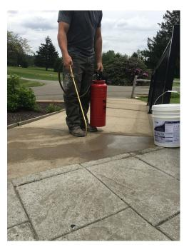
Arisfor<sup>™</sup> Multi-Surface Waterproofer prevents corrosion, spalling and cracks caused by moisture, de-icing salts and chemicals, for new or untreated concrete, masonry and precast applications. The product is suited for home and commercial building facades, parking lots and decks, driveways and curbs, loading docks and ramps, and concrete sidewalks and stairs.
