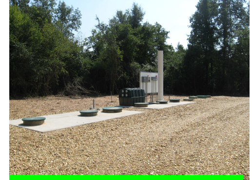
Aerobic treatment + Drip dispersal System.
