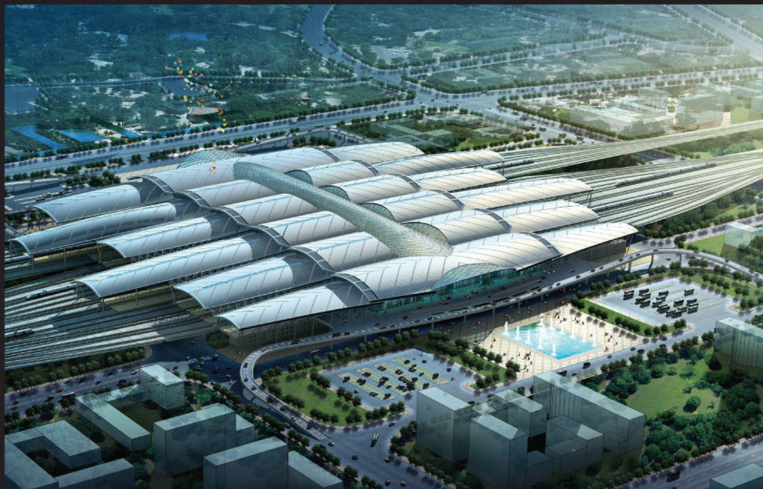
■ (China) GuangZhou South Railway Station
