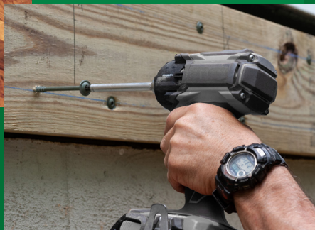
Deck Ledger Attachment
