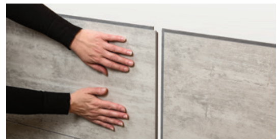
Lock tiles by sliding into joint For wet environments, use a silicone-based sealant in seams.
