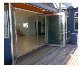
the jamb, while a 60" pivot door with a 12" offset pivot would only project 48". This option creates larger openings with less obstruction.
